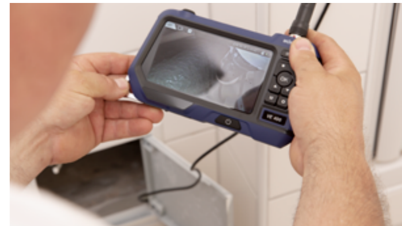
Moisture under the bath? With the Wöhler VE 400, the cause can be found very quickly without having to bring out the "big guns".
